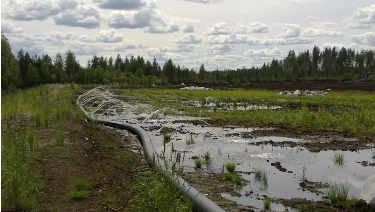
Figure 3. Pumping of run-off waters to the willow plantation at Raatteikonsuo in the summer 2013.
